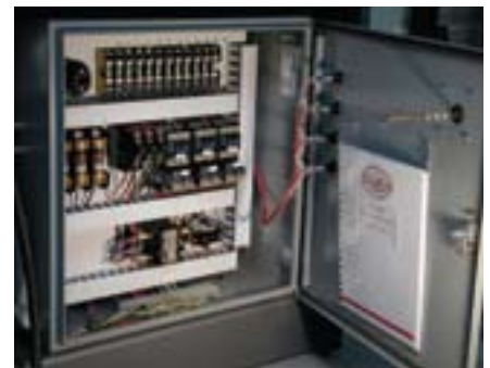
Electrical Box with Operators Manual
